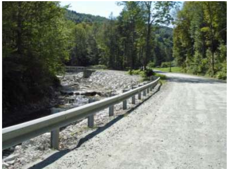
Bethel road after repairs
